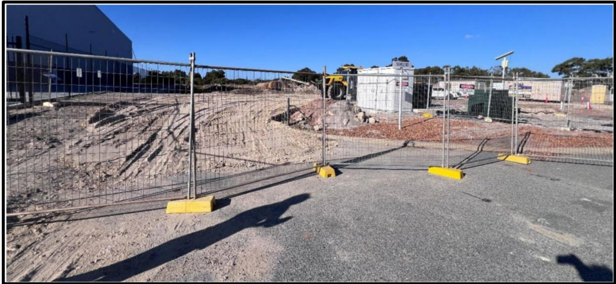
Figure 7-6 Photo of fenced off vehicular access to site on Searle Road
